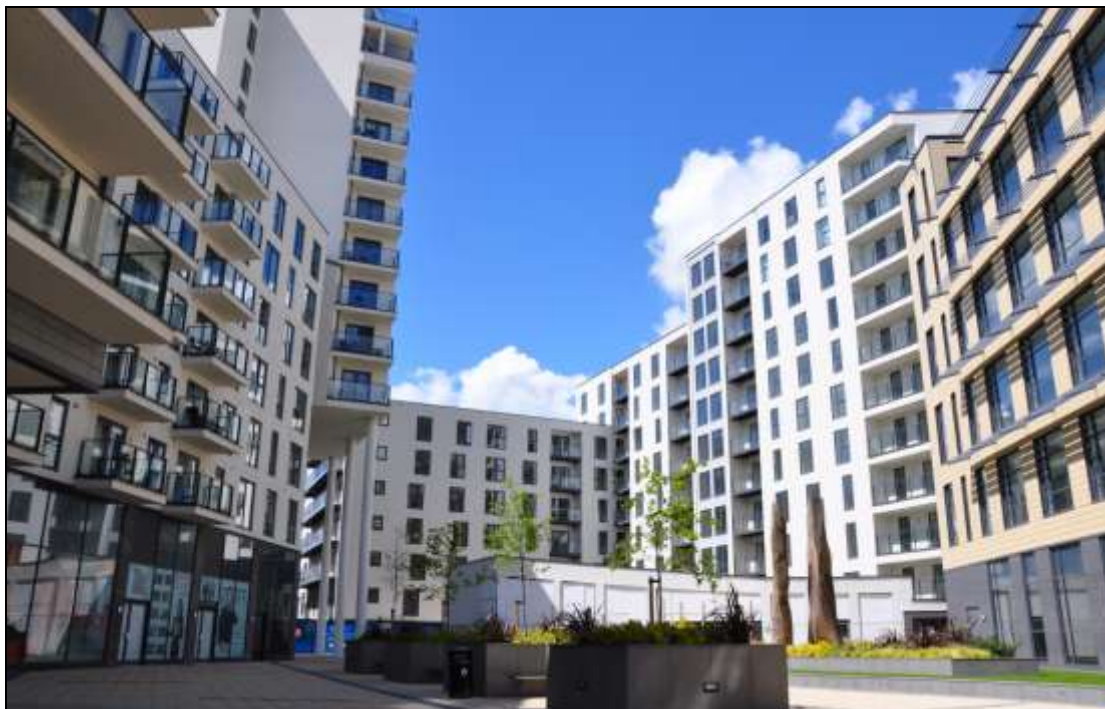
New Central, Guildford Road, Woking Town Centre
